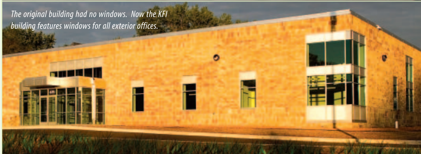
Natural daylighting is provided throughout the facility via these north-facing vertical monitors
